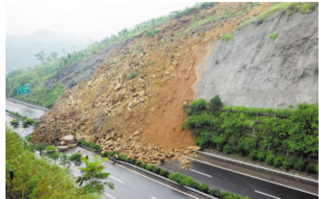
FIGURE 1. A landslide at Yu-Wan highway after completion
