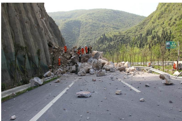
FIGURE 2. A collapse occurred at a handled slope
