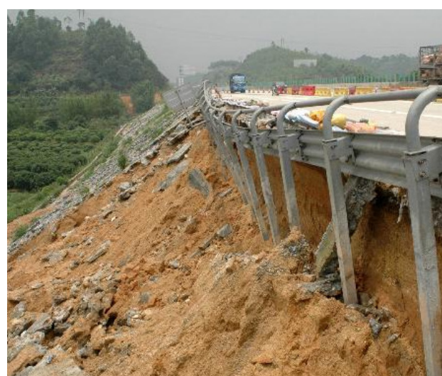
FIGURE 4. A collapse of backfilled slope
