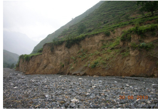
PHOTO 1. A collapse at the study area
