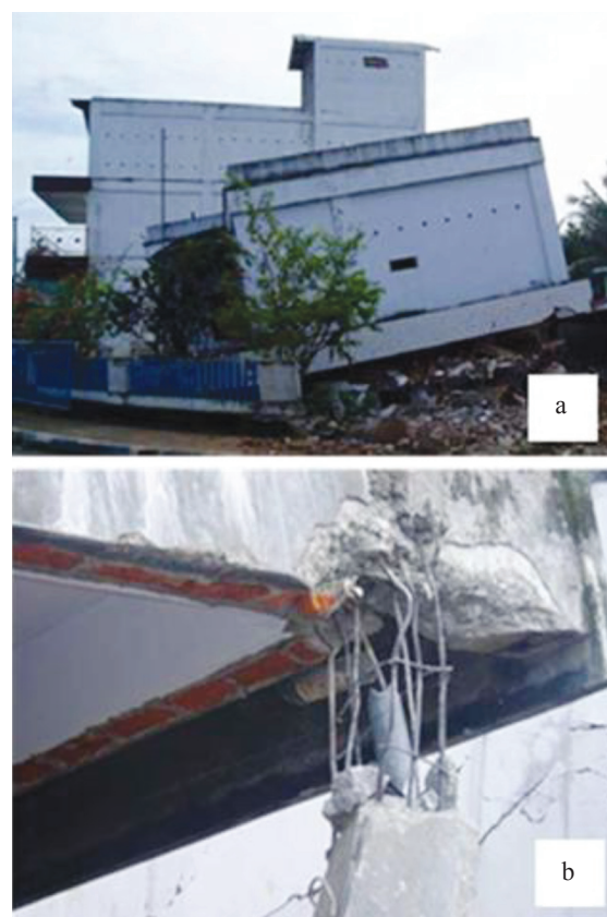
FIGURE 10. Bengkulu Earthquake in 2007, a). The collapsed shophouses, b). Planting utility pipes in the column (source: Boen 2007a).
