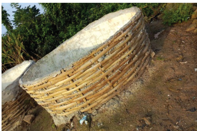
FIGURE 5. Rafter reinforced frustum shaped concrete tank
