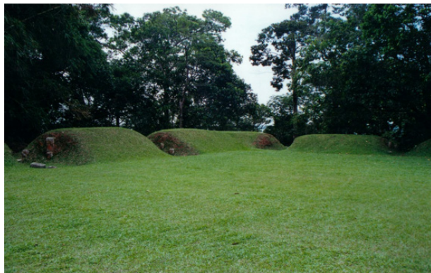
PHOTO 2. Internal view of Kota Johor Lama (Main site) and present condition of walls Source: Asyaari 2012
