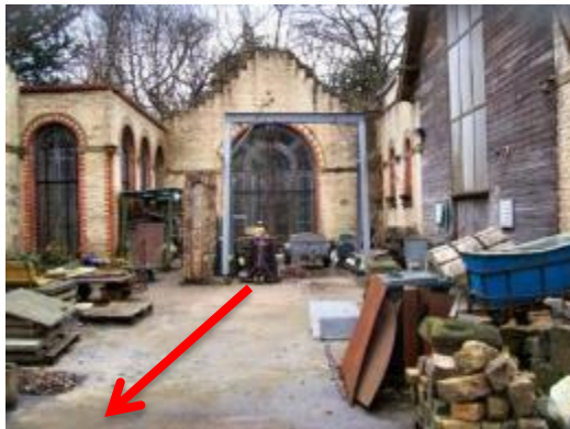
Figure 18: Photograph of the banquet hall interior shows the slope of the exposed floor. Source: (blogspot, 2012).
