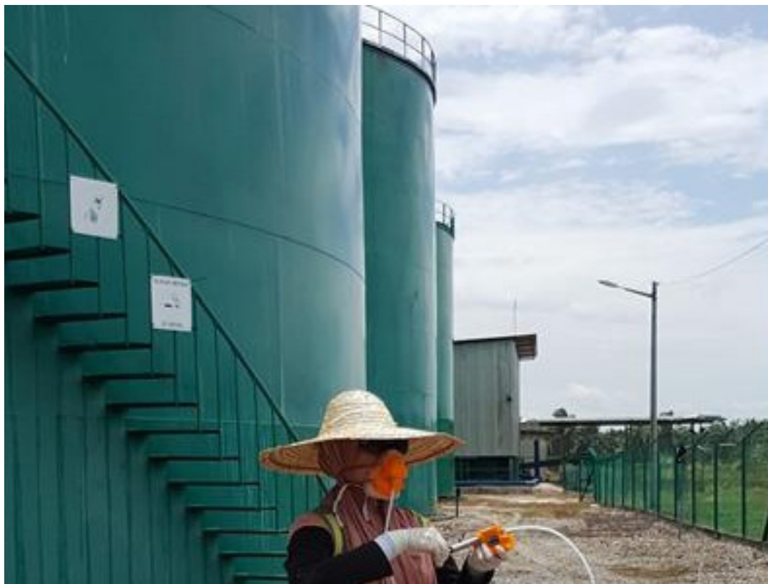
FIGURE 16. Digester tank project site
