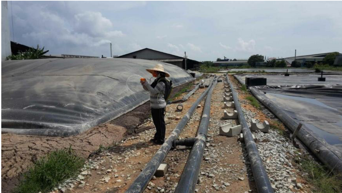
FIGURE 15. Covered lagoon project site
