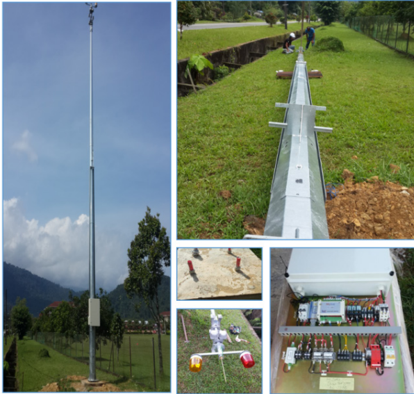
FIGURE 5. EWS installation in Kampung Jenagor
