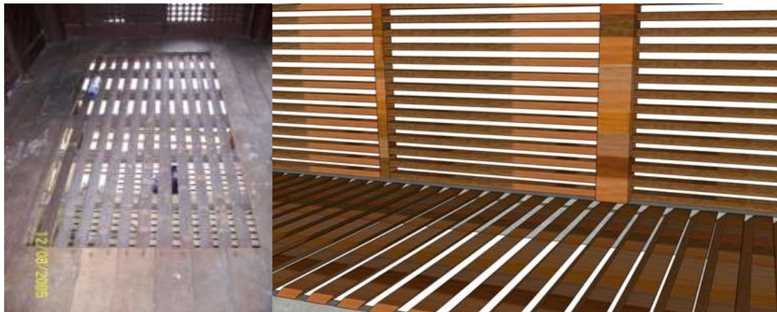
Figure 2 Application of raised floor system with air gaps as evident traditional Malay houses to enable efficient air movement into buildings from under the floor.
