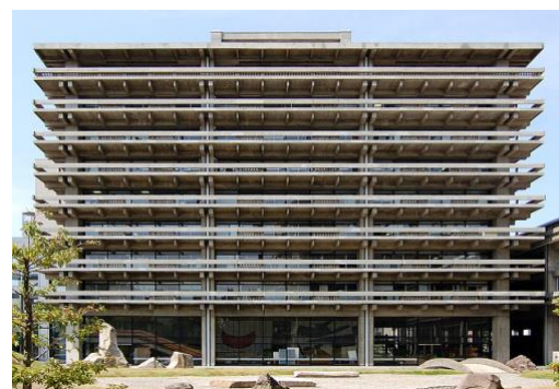
Gambarajah : Kagawa Prefectural Government Office
