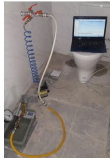
FIGURE 10. Pressure pump to test water pressure
