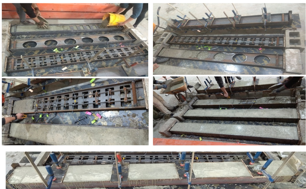
FIGURE 4. Casting of composite specimens using SCC
