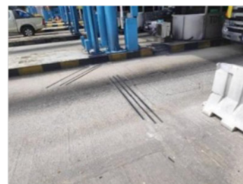
FIGURE 1. The current treadle sensor used at KL-Karak Expressway
