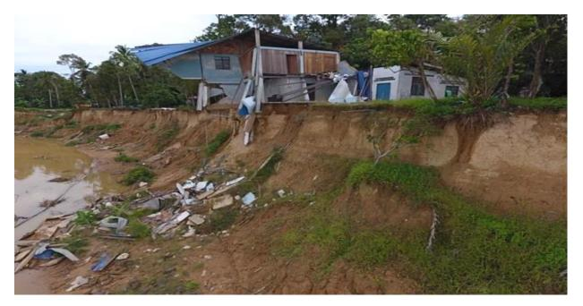
Figure 4. A house that collapsed due to massive river bank erosion
