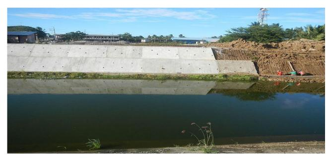
Figure 7. Reinforced concrete to protect the weak river bank
