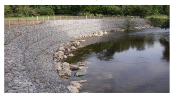
Figure 6. Gabion mattress installed to prevent river bank erosion
