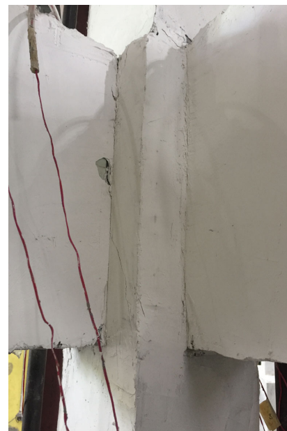
FIGURE 6. Exposure of GFRP sheet and cracks occurred on the specimen due to machine malfunction before the experiment of BCJ with GFRP
