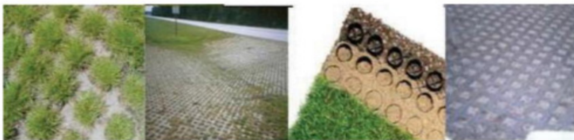
FIGURE 7. Example of permeable pavement/ porous pavement. Source: Garis Panduan Perancangan, Bandar Berdaya Tahan Bencana di Malaysia, 2019.
