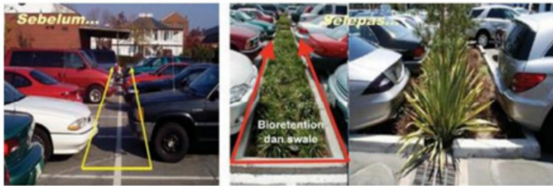
FIGURE 5. Bioretention in the Parking area (TLK) Source: Garis Panduan Perancangan, Bandar Berdaya Tahan Bencana di Malaysia, 2019.
