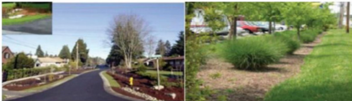
FIGURE 6. Bioretention along the roadside. Source: Garis Panduan Perancangan, Bandar Berdaya Tahan Bencana di Malaysia, 2019.
