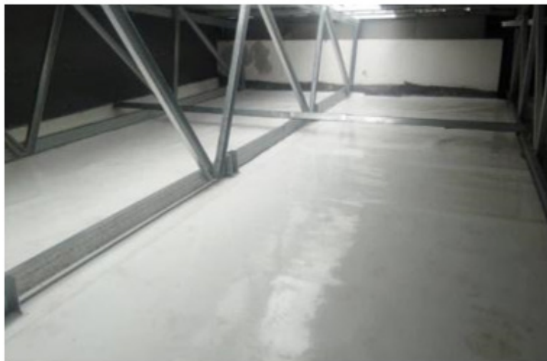
FIGURE 12. Single-ply membranes are installed under the metal roof
