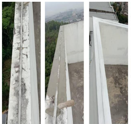
FIGURE 8. Repair work of a wall adjacent to the lift motor room.
