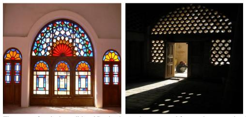
Figure 8. The porous facade, in traditional Iranian house that, was used for creating more visual privacy and with ability to have visual access from inside to outside and decrease visual access from outside and decreasing the temperature
