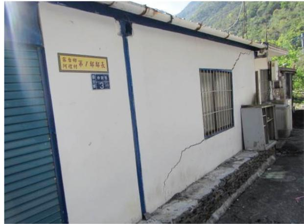
FIGURE 9. Landslide caused damage in Ali village
